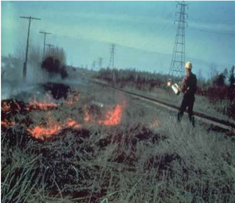
Figure 7.81. Right-of-way maintenance burning.
