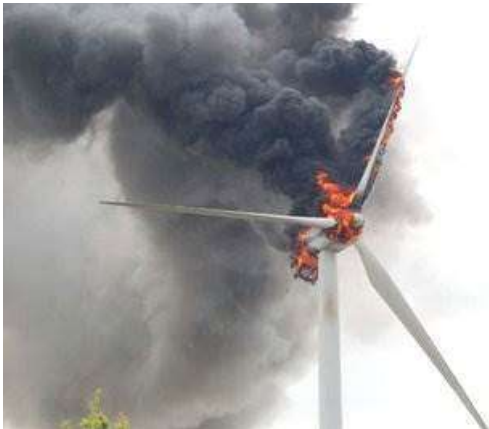
Figure 7.71. Wind turbine fire.
