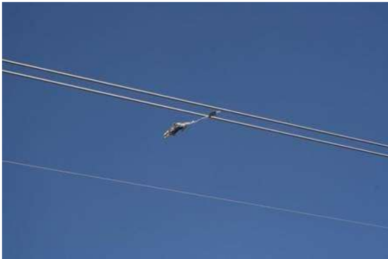
Figure 7.46. Mylar balloon stuck on transmission lines.
