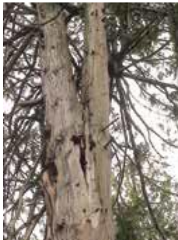
Cedar with open cracks.
