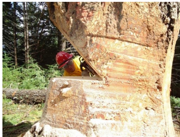
The sloping cut is at a 45-degree angle.
