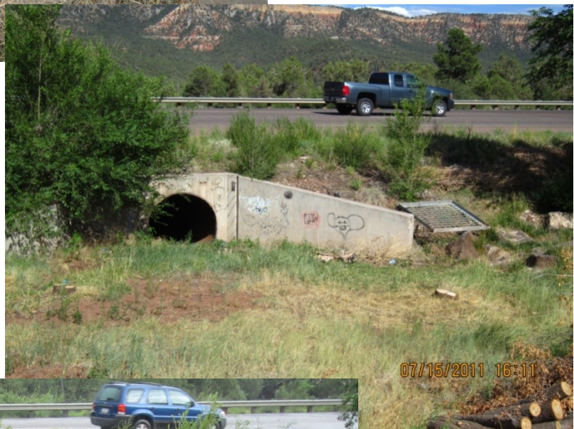
Culvert under Highway 73 at Mulberry Ave.
