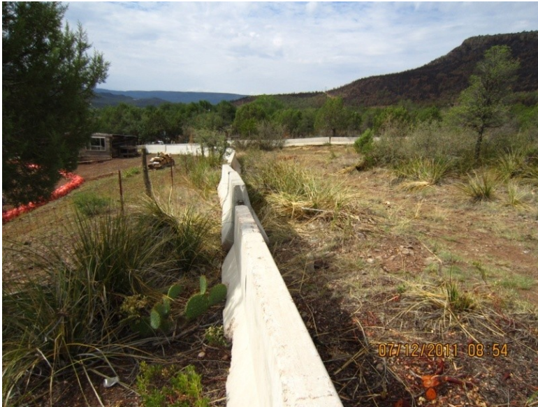
Behind k-rail right after installation
