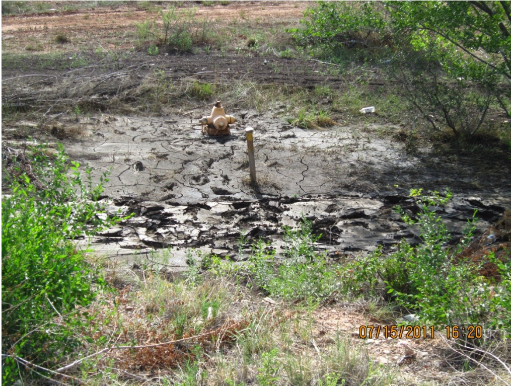
After first small storm: Notice pipe and cap in foreground. Before fire the hydrant was fully visible.
