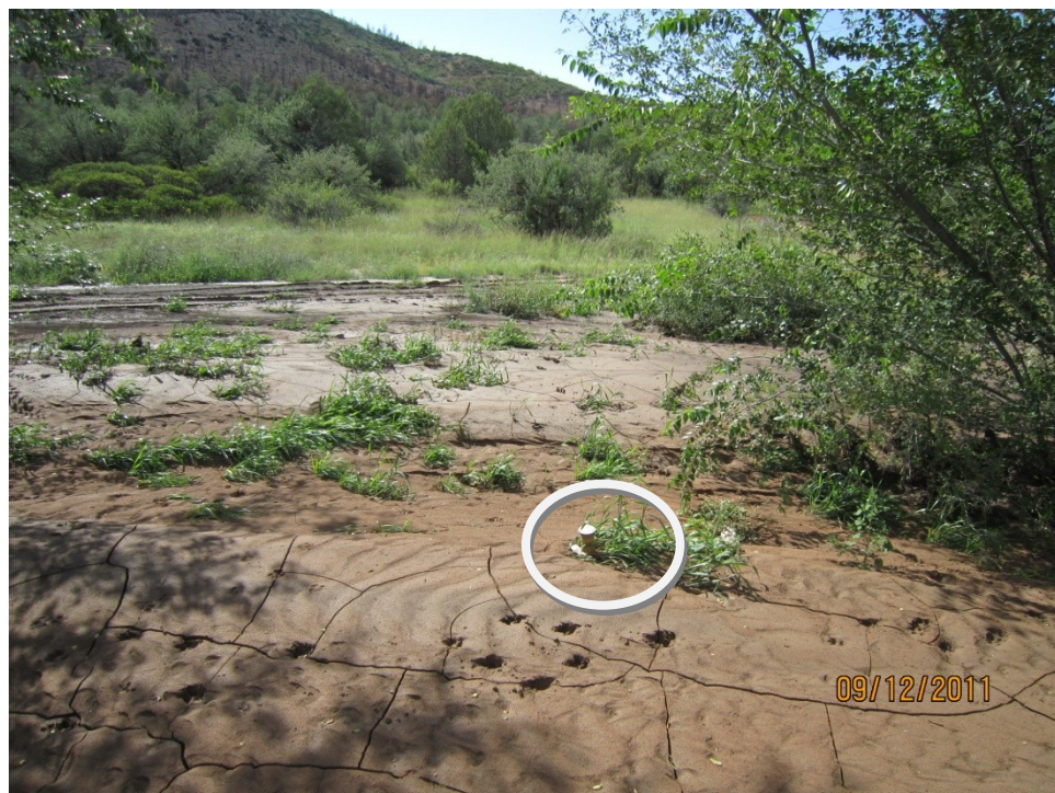
Same location after 4 th storm: Note pipe and cap in foreground..but missing fire hydrant under the mud.
