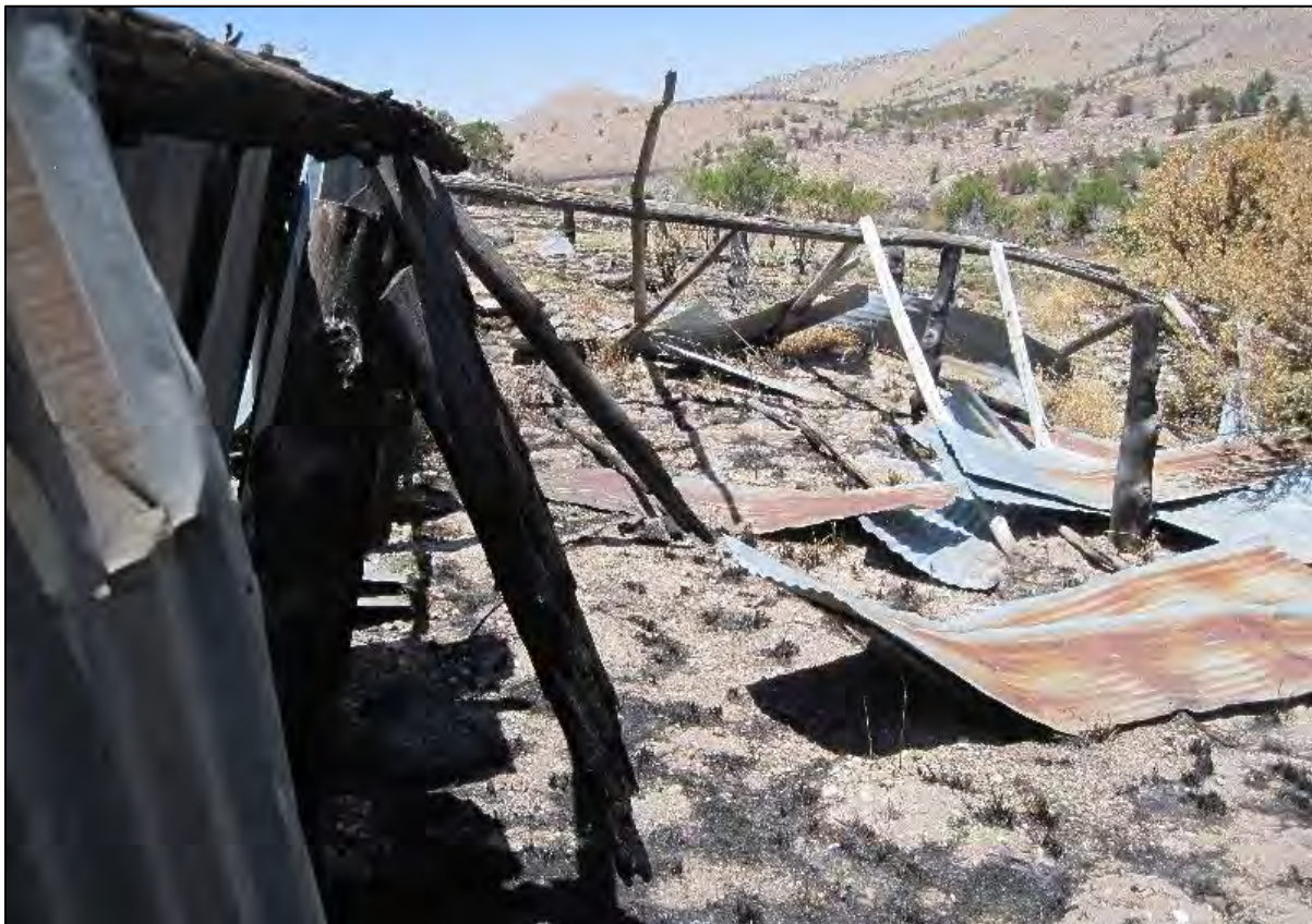
Figure 45: 41CU150 burned wall supports in barn.
