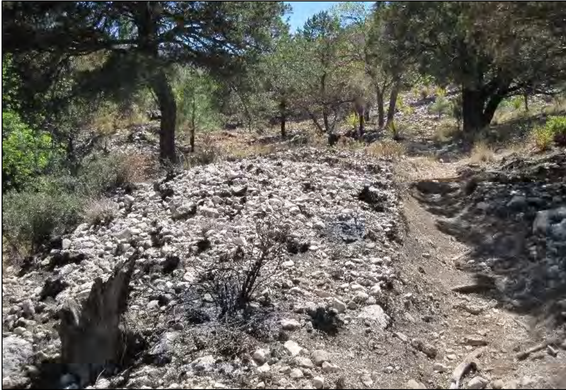
Figure 22: 41CU96 Feature F3 facing west with trail destruction.
