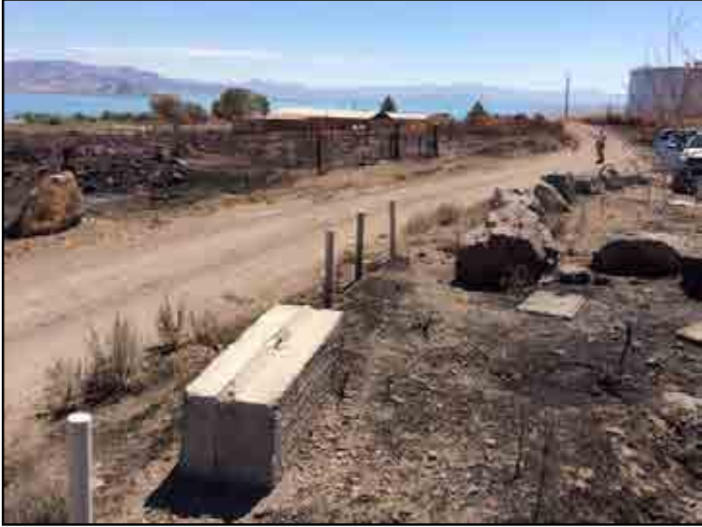
Dunn Hatchery at Risk from Flood and Debris Flows from Hardscrabble Creek
