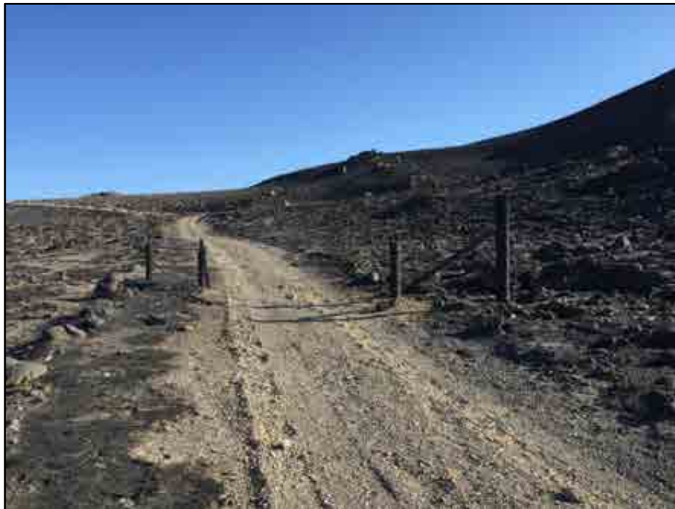
Fire Damage to End Panels and Gate
