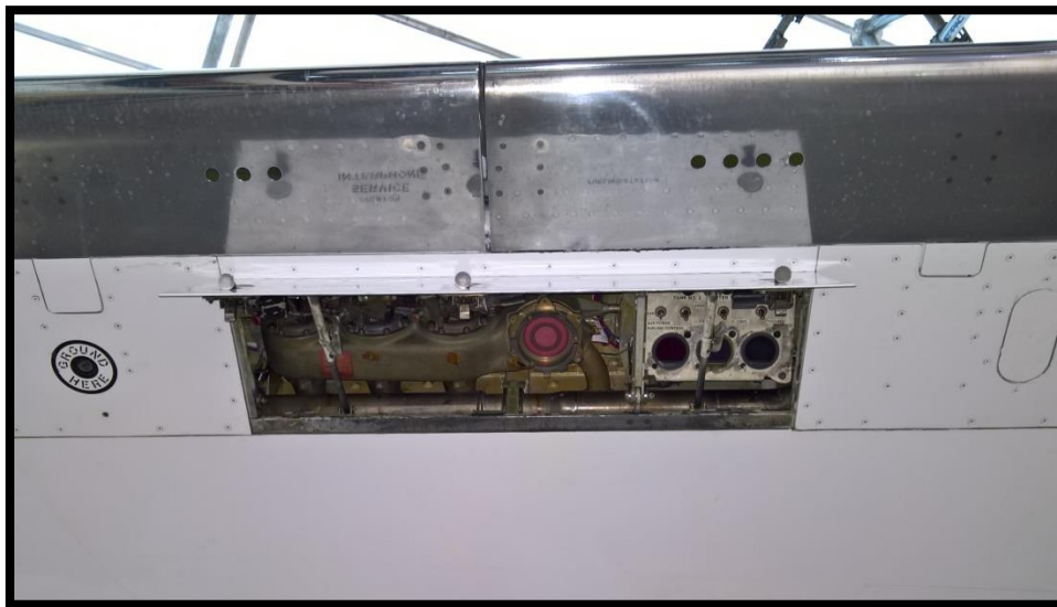
Figure 15 Boeing 737 Single Point Fueling Station (Open)
