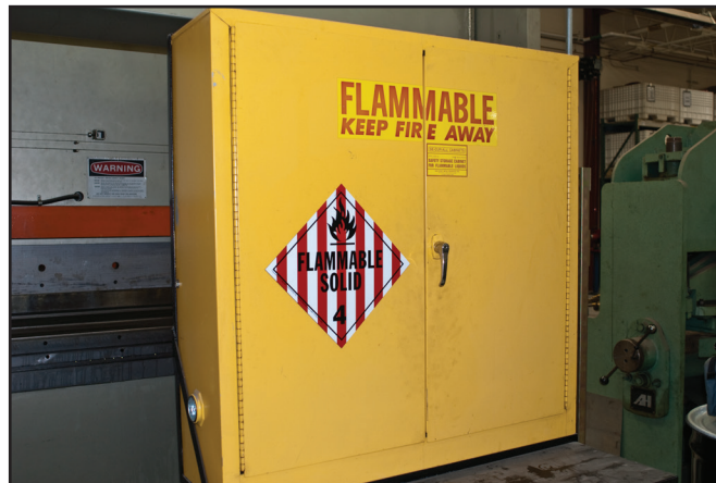
Figure 4-15—This cabinet is labeled properly for storing flares.
